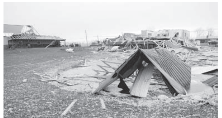
Severe storm damage to homes is seen on Plymouth Springmill Road just south of the intersection of Ohio Route 96 in Shelby, Ohio, Sunday, April 14, 2019.
